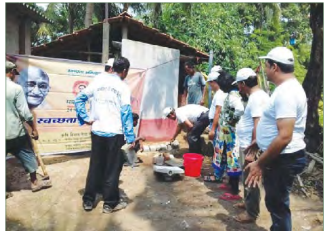
Construction of low cost toilet
